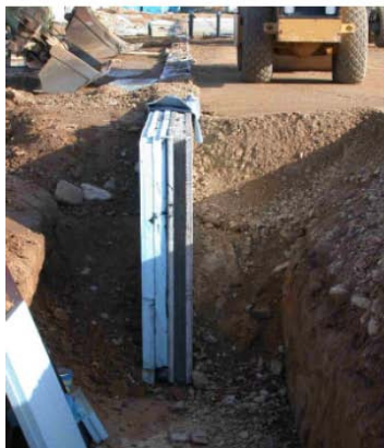
Construction of the frost barrier and the rear ventilated façade
