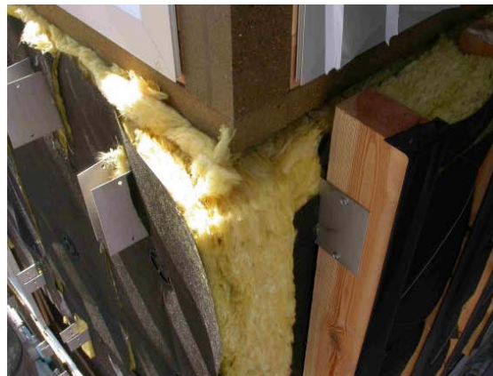
Construction of the frost barrier and the rear ventilated façade
