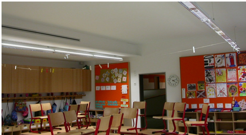
Classroom with suspended ceiling, acoustic bulletin board, dispersion slot (fresh air), certificates
